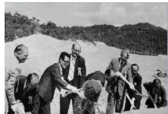
Groundbreaking ceremony for KRIS (1976)
